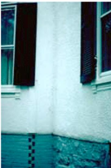
If the test samples are not executed on the building, they should be placed next to the stucco remaining on the building to compare the color, texture and composition of the samples with the original. The number and thickness of stucco coats used in the repair should also match the original.
